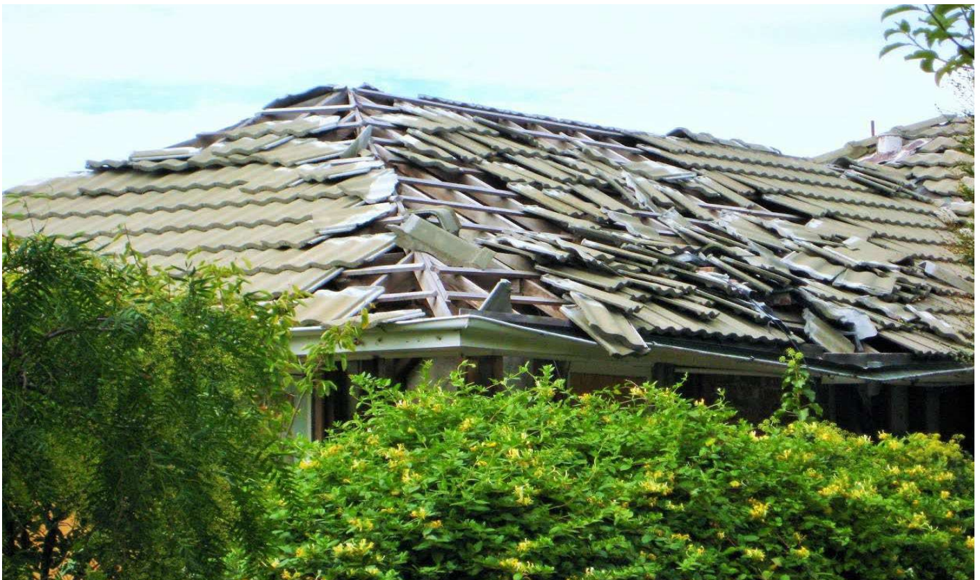
Figure 1: Christchurch. Earthquake damage. Source: Louise Thornley
