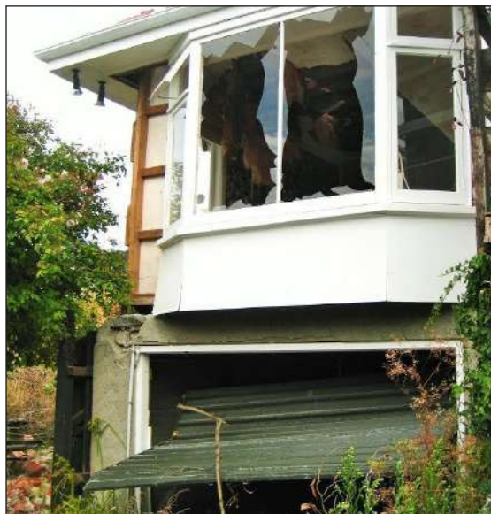
Figure 32: Christchurch. Earthquake damage. Source: Louise Thornley
